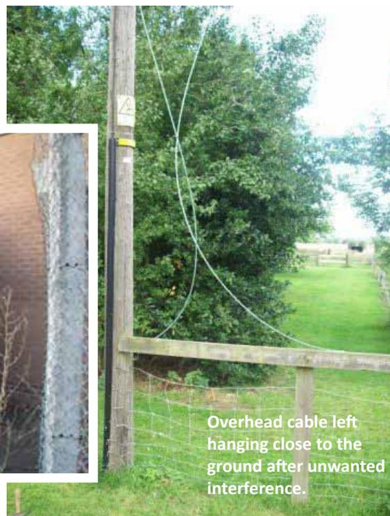
Overhead cable left hanging close to the ground after unwanted interference.
